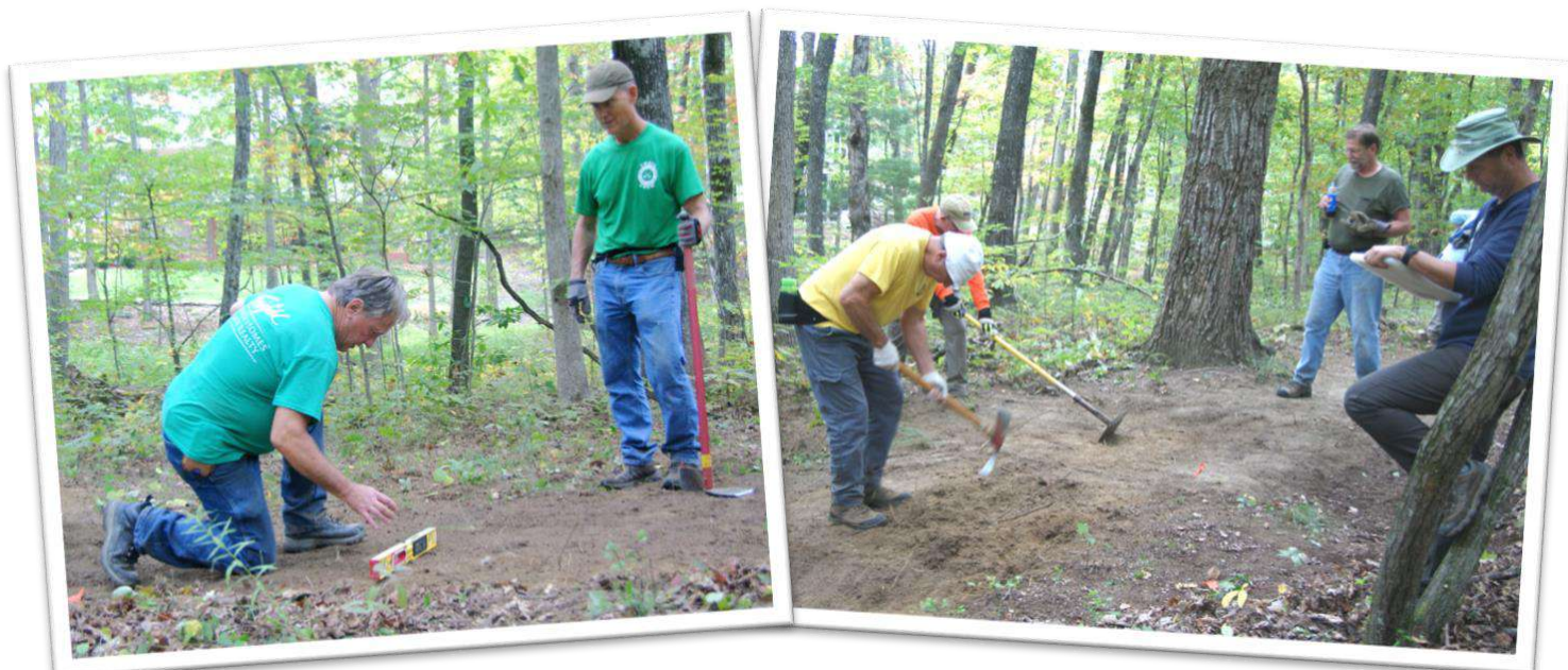
Left: Dale Butson uses a digital level to check the out slope of the trail tread just built by Pat Gundy.
