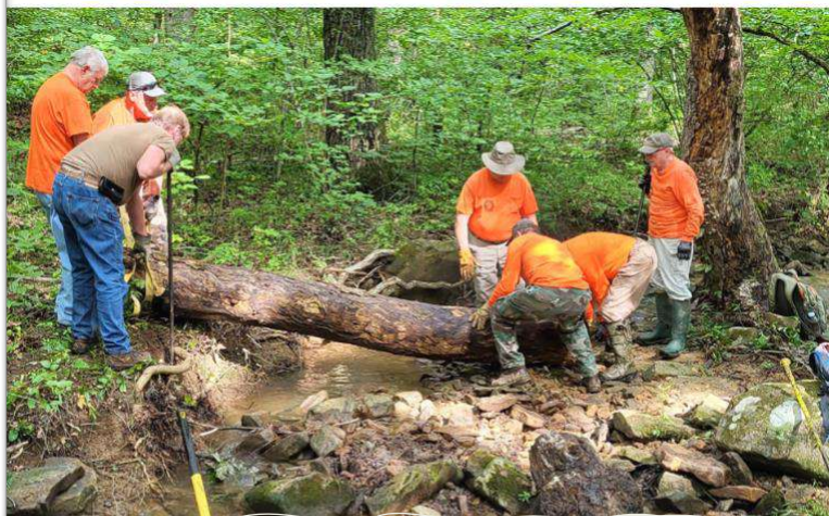
The Trail Crew needed to clear a large dead fall in the creek by Bridge 7 of the Seven Bridges Trail. The tree changed the water course and began to undermine the bridge. It took several rock bars and six people to manhandle it out of the creek bed.
