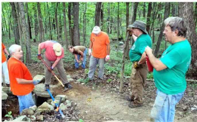
In preparation for the Marathon, the Trail Crew made repairs on the Canyon Trail, because water runoff from Chestnut Ridge is a continuing problem. Nearly 100 feet of trail was rebuilt and a deep channel dug to keep the water off the trail.
