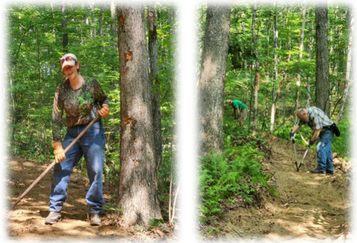
Sue Heritage performs slope work (left) while Don Eller and John Partyka (right) lop roots on the Airport North Loop in Crossville.
